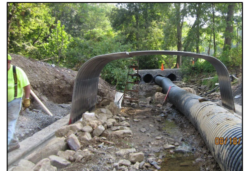
Assembly of a 15' w x 6' h bottomless arch pipe on cast-in-place footings (Juniata).
