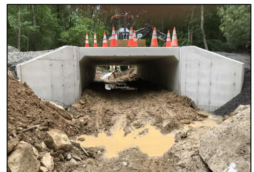
Bottomless concrete box culvert (Cumberland)
