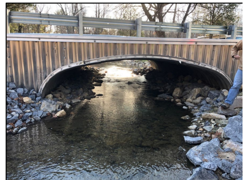
19' w x 6' h structure showing low flow channel and bank margins (Northampton)
