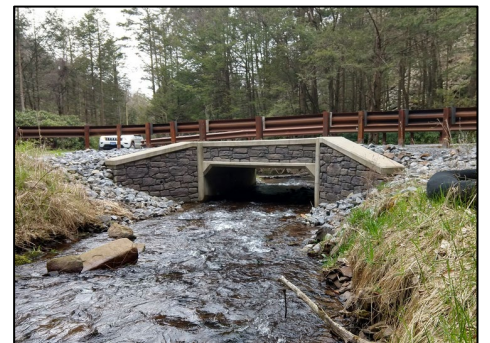
Concrete box with stamped concrete headwall (CDGRS).
