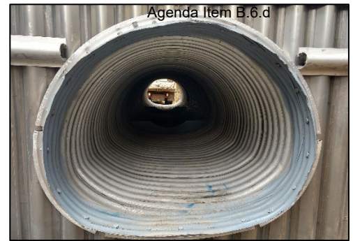
Pipe arch or "squash pipe" (6' wide) (CDGRS)
