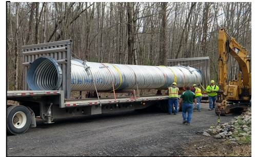
Delivery of a fully assembled 6' w x 4' h x 40' l pipe arch (CDGRS).
