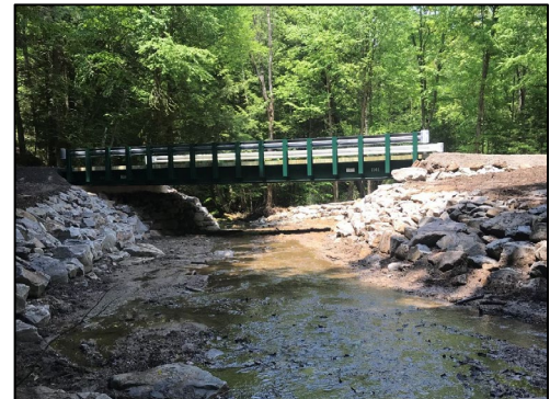
Completed 50' span (~25' channel) spread footer bridge (Indiana).
