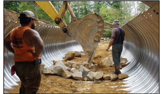
Photo 2: Placing large material during pipe assembly.
