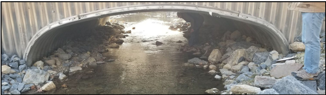
Figure 1.1 Example Stream Crossing
