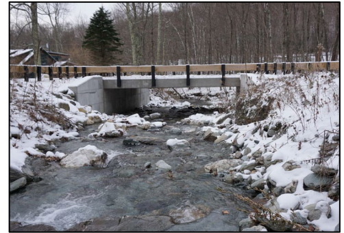
Traditional 22' precast concrete deck bridge on poured-in-place concrete footings (TU).
