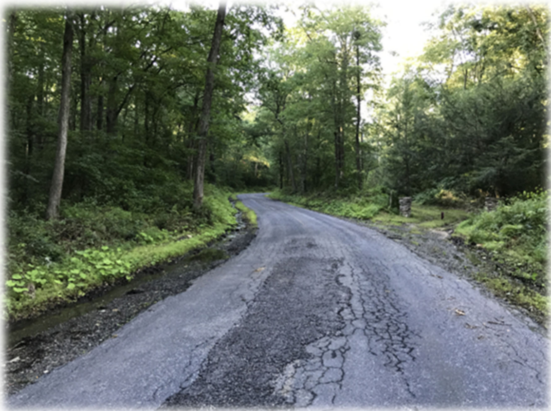
Before picture of cover photo project. 800 feet of underdrain and a 500 foot French Mattress served to dry out this saturated roadbed. Paving was done in-kind.
