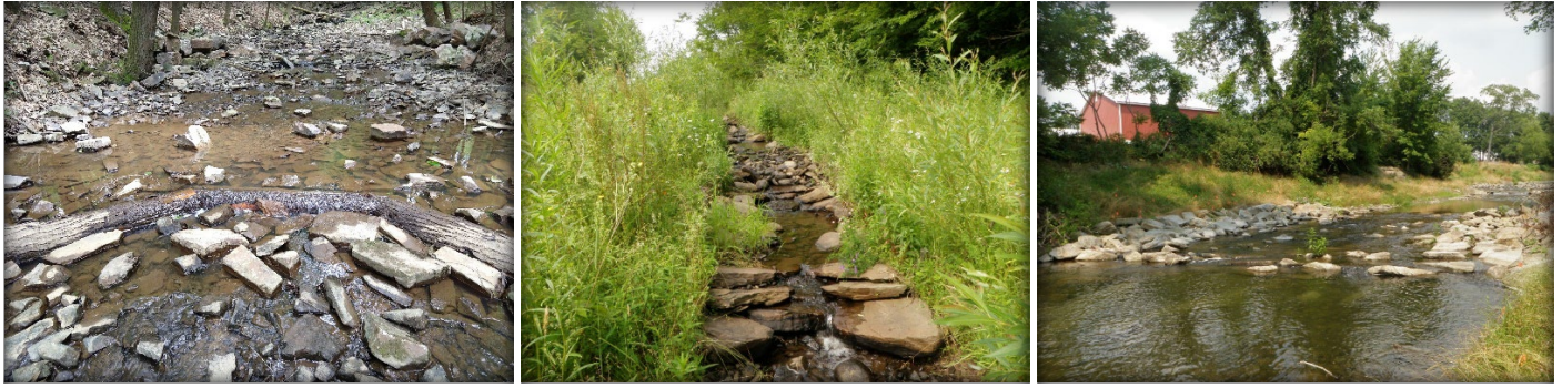
Figure 1: From left to right, log cross vane with throat log, rock clusters and cascade, and constructed riffle.
