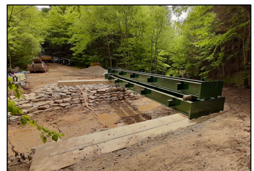
Spread footer bridge installation (Indiana)
