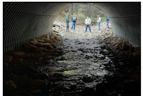
Completed 16' w x 10' h pipe arch (Crawford).
