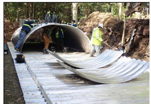
Assembly in-place of a 12' w x 5' H pipe arch (Elk)
