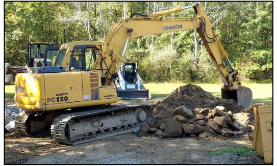
Photo 5: Mixing native material and larger foundational stone prior to placement.
