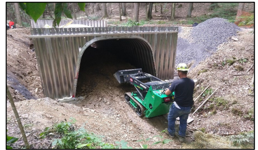
Photo 2: Placing fine material in a 8'w x 6'h bottomless arch with a walk behind skid steer.
