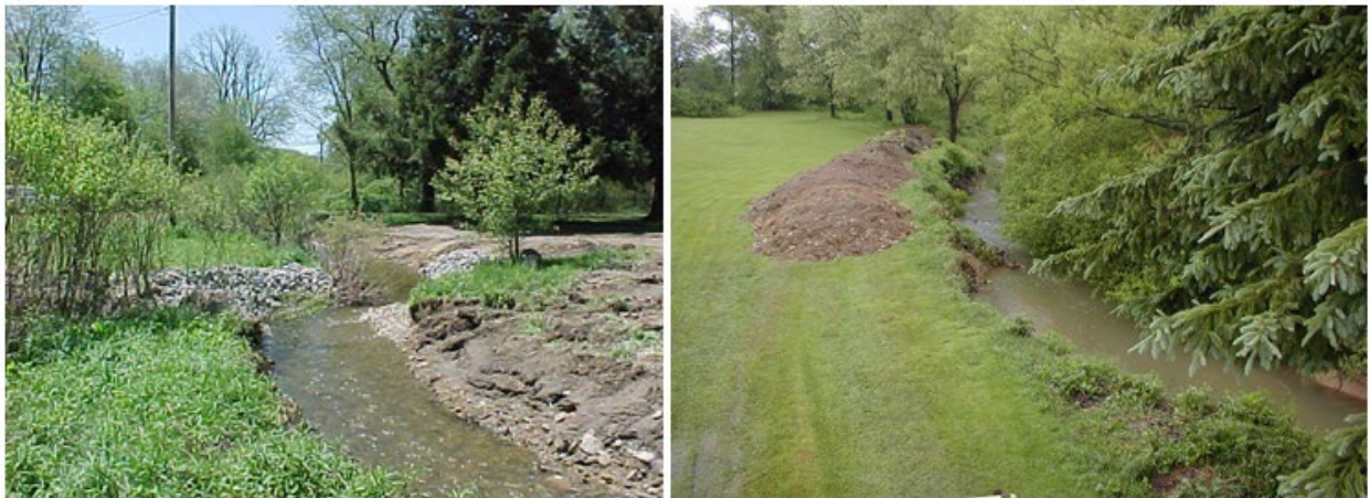
(Left): A pile of fill consisting of rock or stone is encroached into the stream channel. (Right): A pile of fill consisting of soil is located in the floodway and poses a water obstruction . In both cases, these activities may require a permit under Chapter 105 regulations. Credit (both): PA DEP
