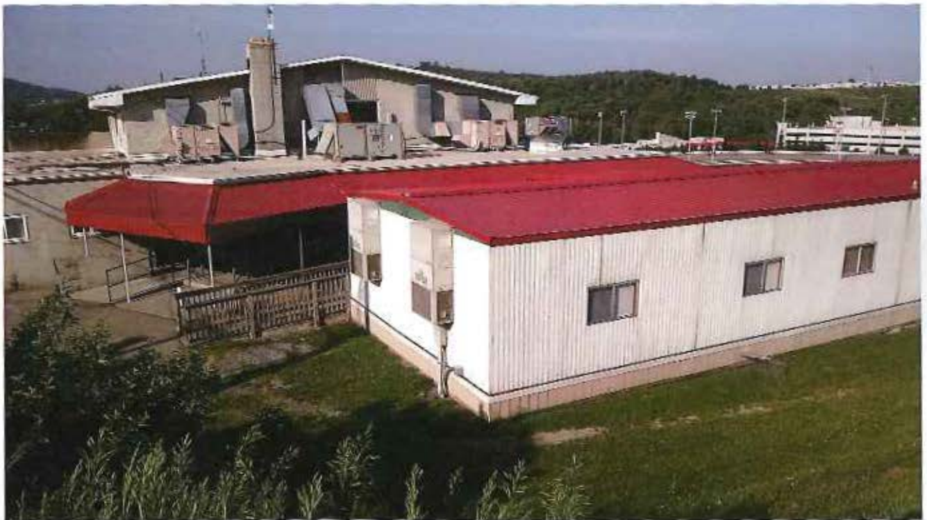
New roof and awnings on race office and horsemen's trailer
