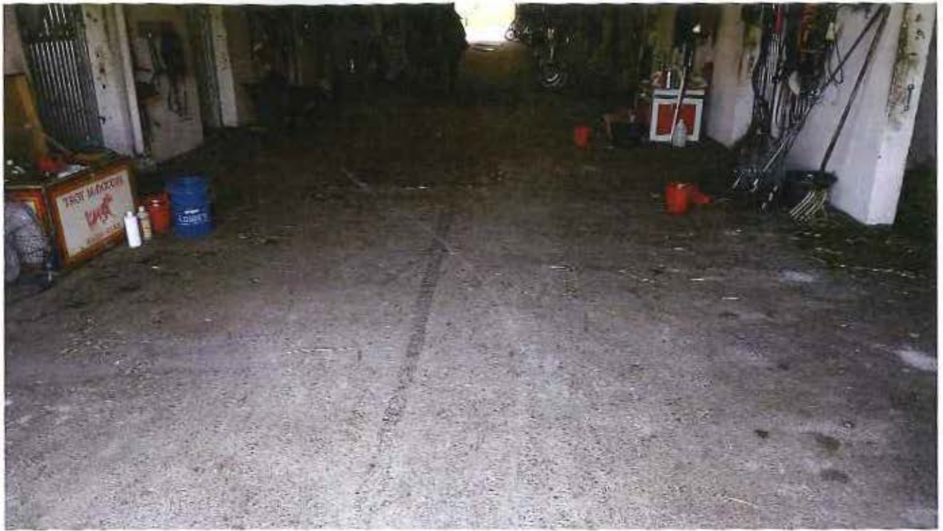
Newly paved aisleways in the barn area
