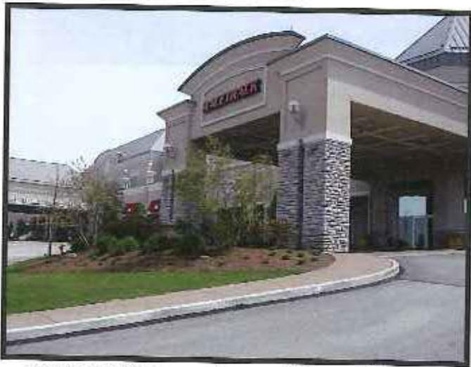
Racetrack Entrance from outdoor parking area
