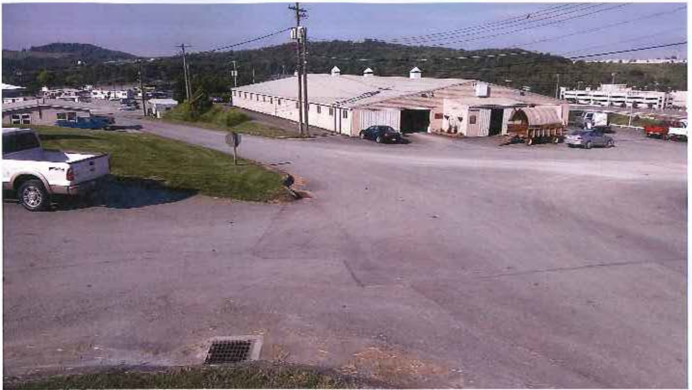
Repaved roadways throughout backstretch
