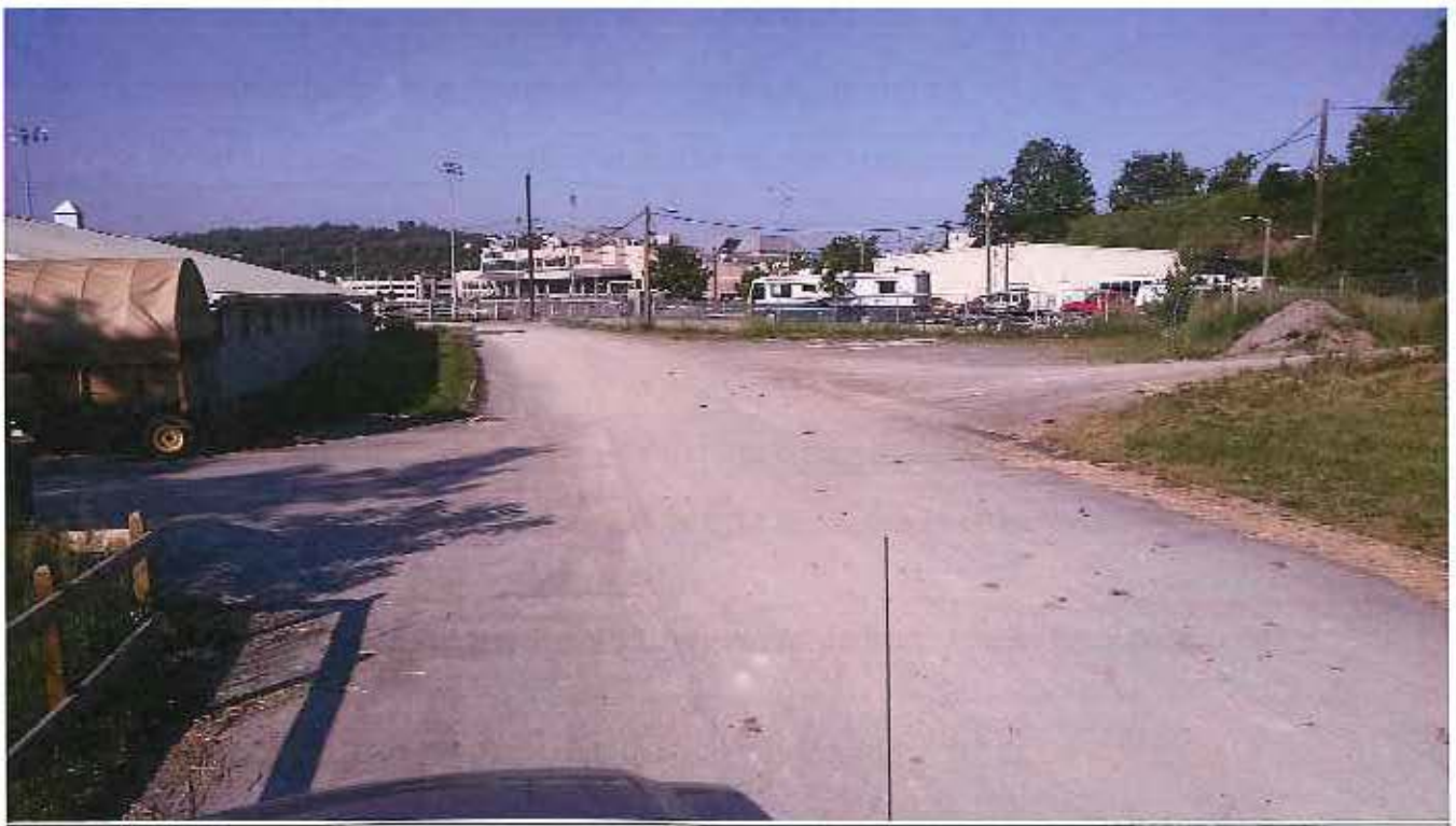
More repaved roadways
