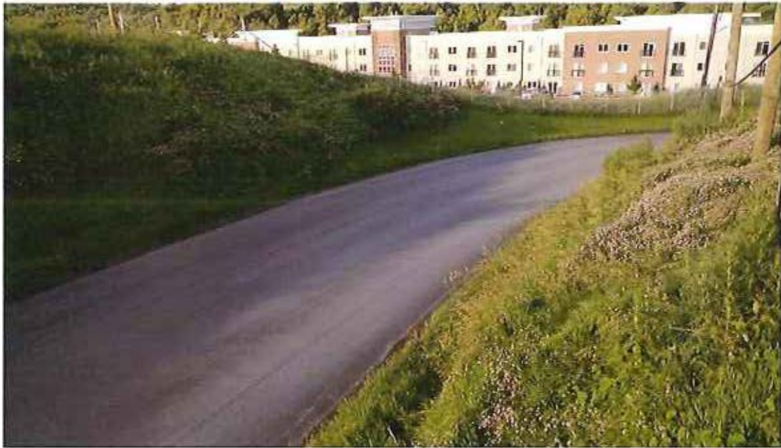
More repaved roadways
