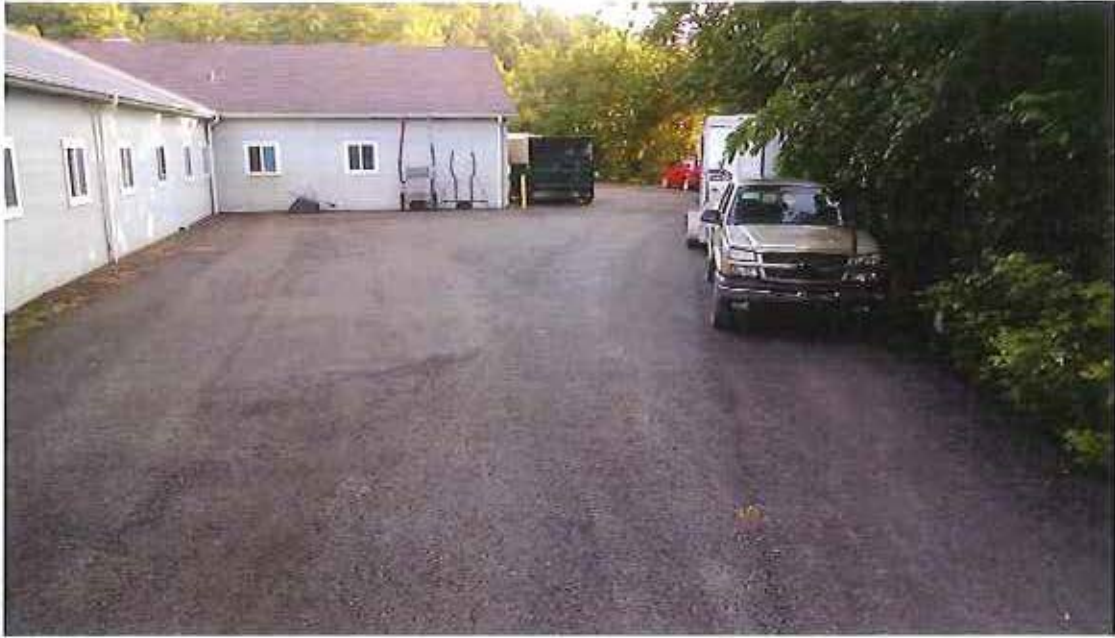
Repaved roadways throughout backstretch
